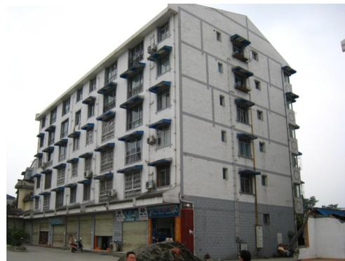
Fig. (2). Typical confined masonry buildings in Sichuan.
