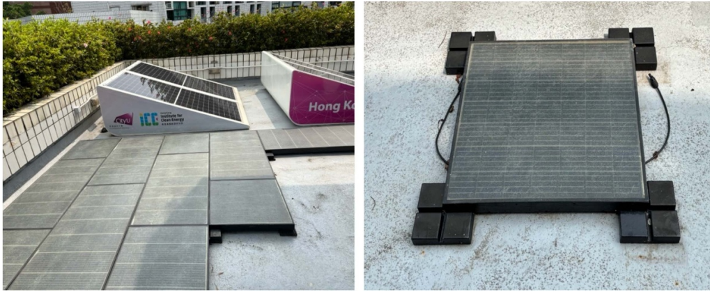
Figure 3. Solar pavement at Hong Kong Institute for Clean Energy (HKICE) at City University of Hong Kong.
