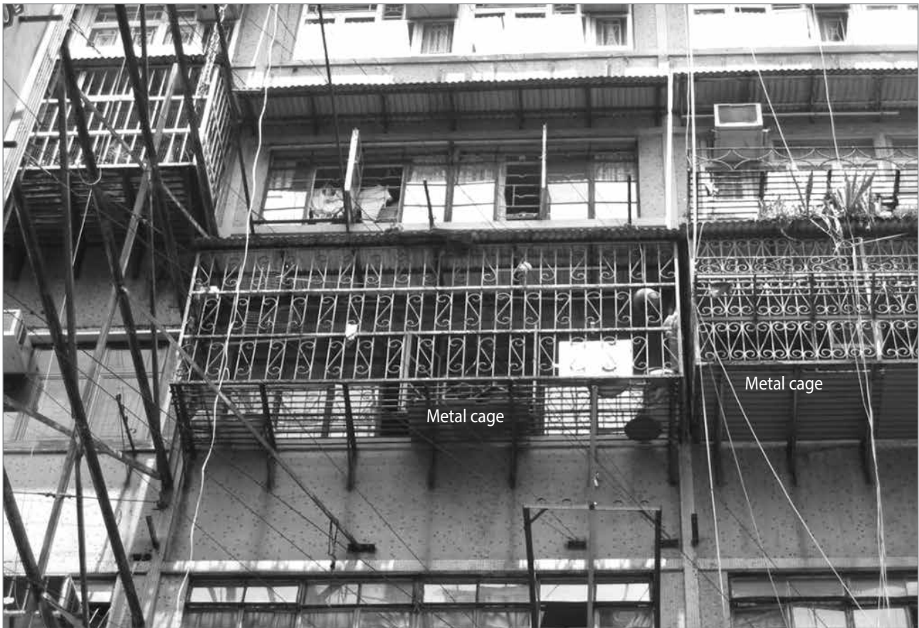
Figure 3: Metal cages (photo: Yung Yau).
