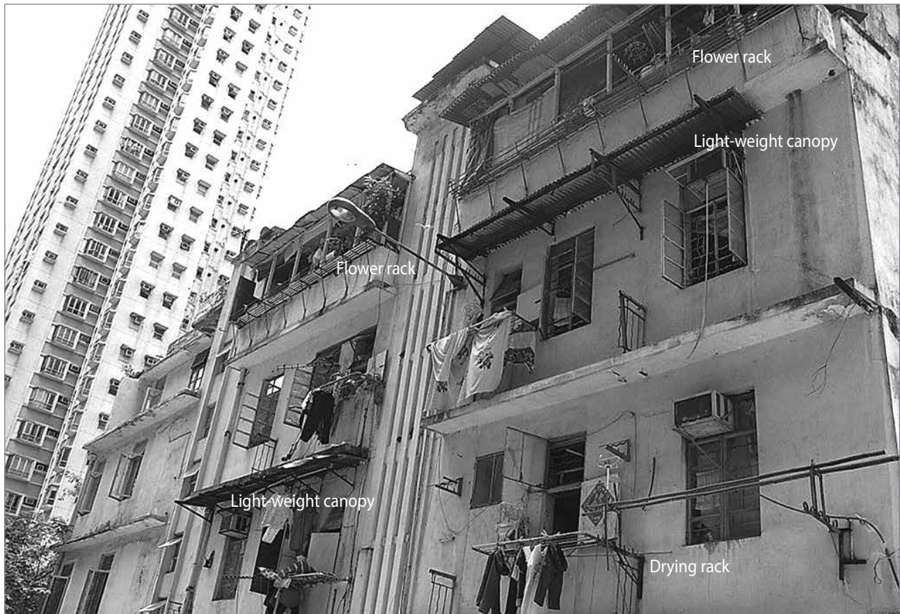
Figure 1: Lightweight canopies, flower racks and drying rack (photo: Yung Yau).
